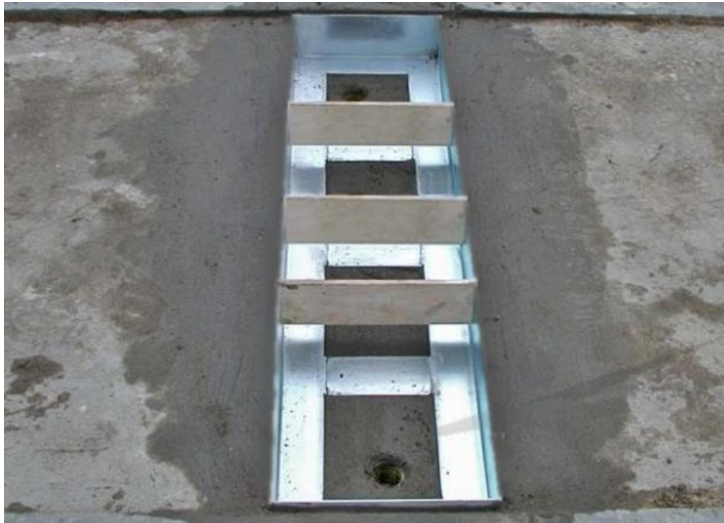
Image 1. Installed tray secured with spacing boards
