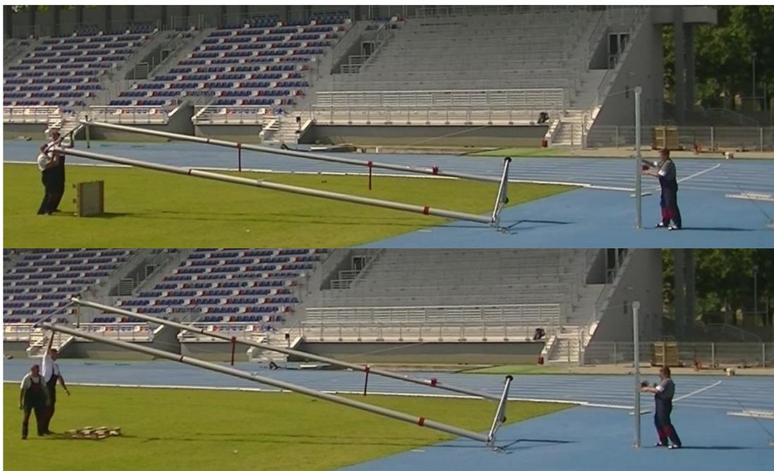
7. After the gate is lifted, fix the extreme pillar to the anchor.
