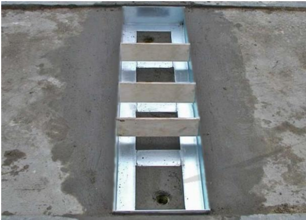
Image 1. Installed tray secured with spacing boards
