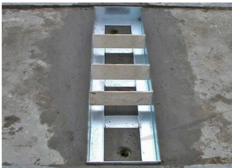
Image 1. Installed tray secured with spacing boards
